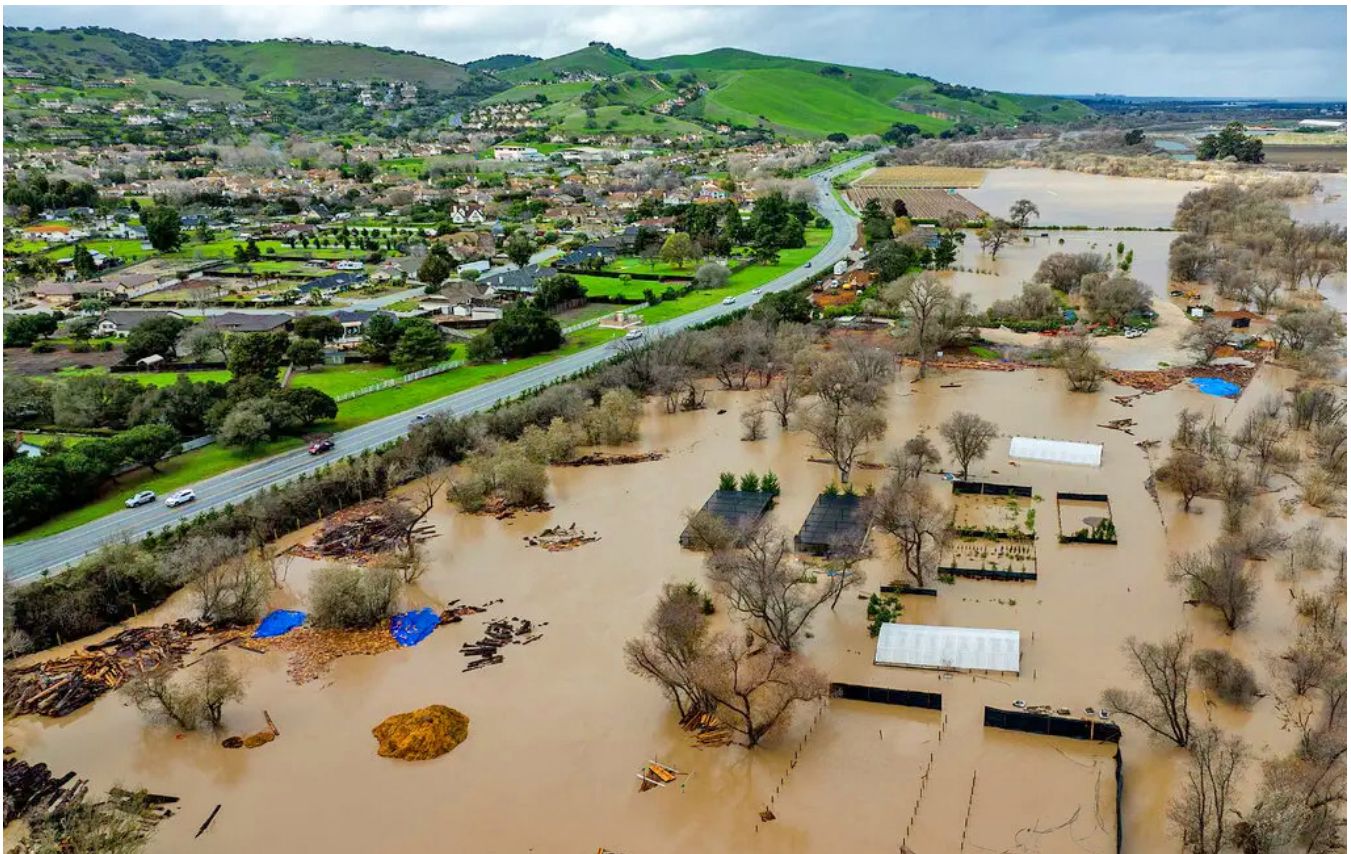
A 2021 winter storm causes stormwater flooding.
