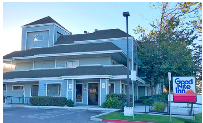
Through Project Homekey, the City received $9.2 million to acquire the Good Nite Inn and transform it to 101 units of permanent supportive housing.
