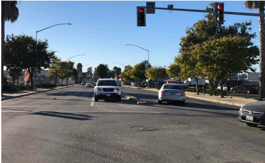
The existing roadway configuration at Work Street (looking west) includes four travel lanes, one turn lane, and curb-side bike lanes on both sides.
