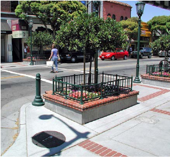
Sidewalk extensions shorten crossing distances and provide room for additional pedestrian amenities.
