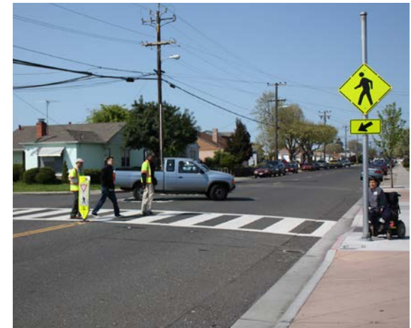
Crosswalk enhancements can include high visibility signage and striping.
