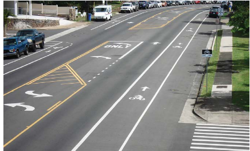
As seen in this example, the west segment concept includes two travel lanes and a center turn lane. However, as shown in Figure 4.3, the concept includes a buffered bike lane and no on-street parking.
