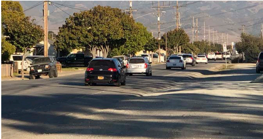
The existing roadway configuration near Market Street (looking east) includes two travel lanes, on-street parking on the north side, an unpaved shoulder on the south side, and curb-side bike lanes on both sides.
