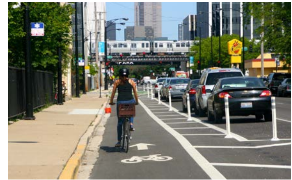
This protected bikeway is separated from vehicle traffic by painted buffers, flex posts, and parked vehicles.
