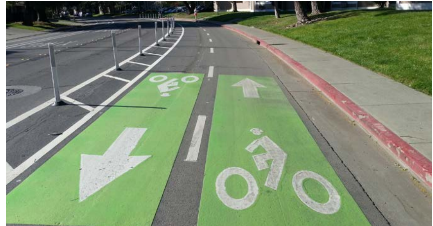
Two-way cycle track separated from the street by a painted buffer and flex posts.
