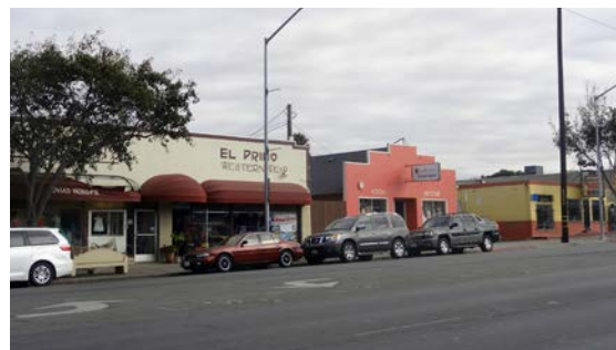
The majority of commercial buildings along the central corridor are of older construction, single-story, have brick and stucco facades, and have minimal architectural detail.
