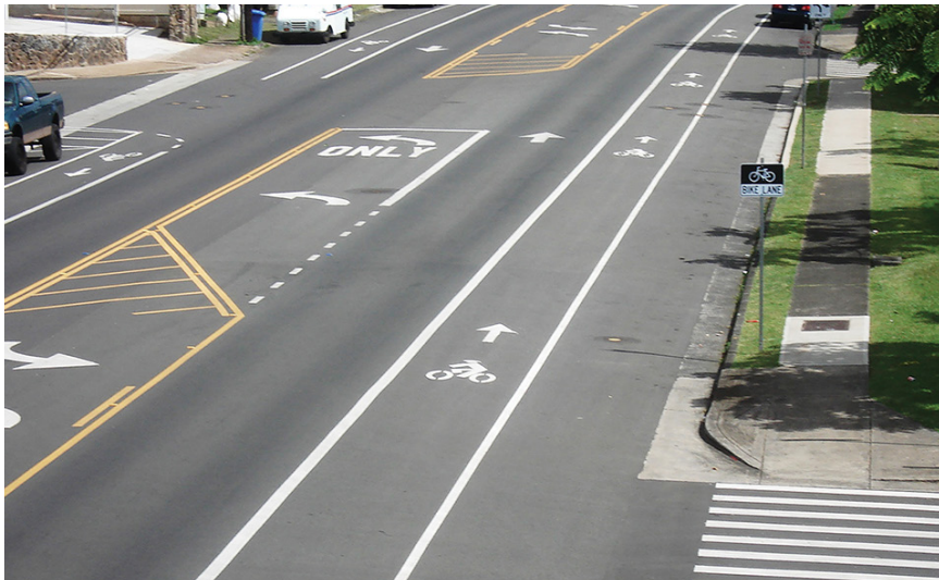
This image shows a roadway with two vehicle through lanes and a center turn lane, allowing sufficient width for safe bicycle facilities.
