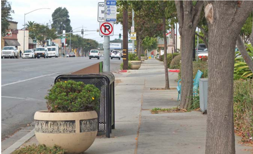
This sidewalk near Madeira Street is functionally narrowed by utilities, tree wells, and other features placed in the travel path.
