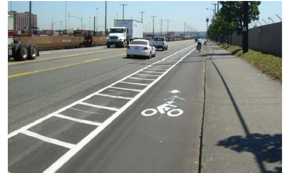
The west segment proposed improvements include buffered bike lanes on both sides of the street.
