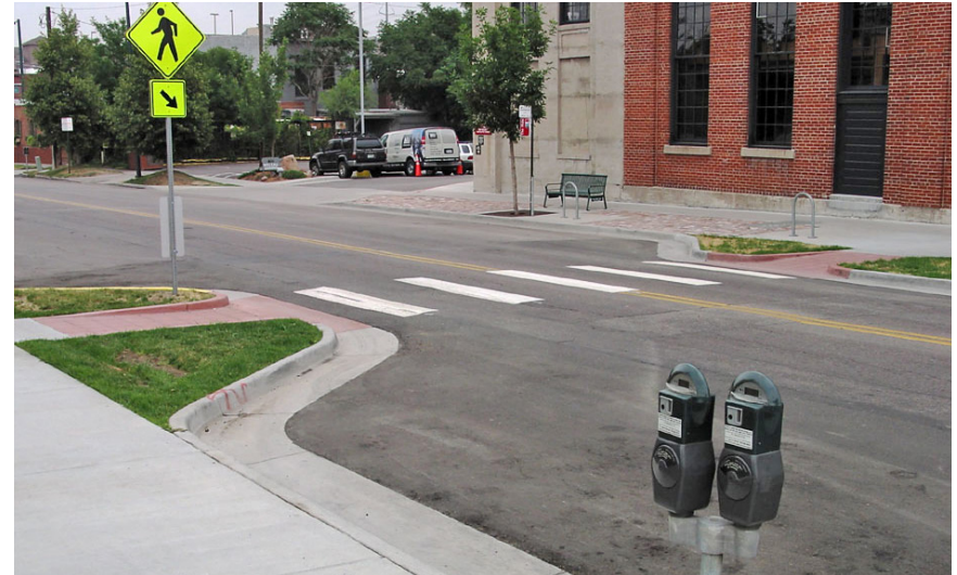
Sidewalk extensions narrow crossing distances, improve pedestrian sight lines for drivers, calm traffic, and provide space for additional amenities and landscaping.
