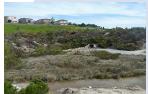
Supplemental detention / retention basins designed to have a natural vegetated appearance.
