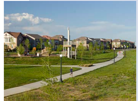
A network of enhanced pedestrian paths that link the neighborhoods is well represented in the West Area Specific Plan.
