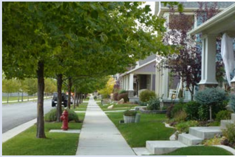
Recessed garages and reduced front yard setbacks provide pedestrian-oriented local streets and reflect CPTED principles of “eyes on the street”.
