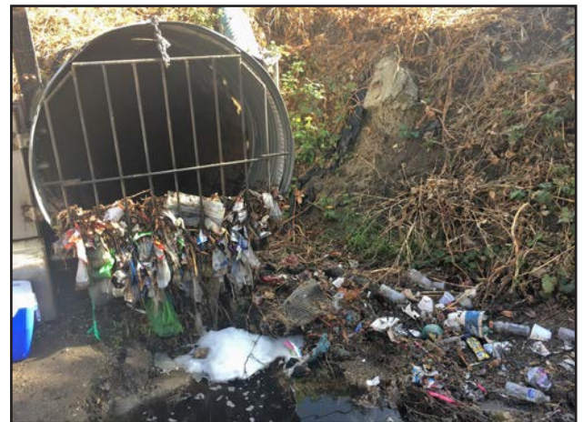
Same terminal outfall on First Flush 2017 (11/2/17) after 0.13in of rain. More than 130 gallons of trash were collected.
